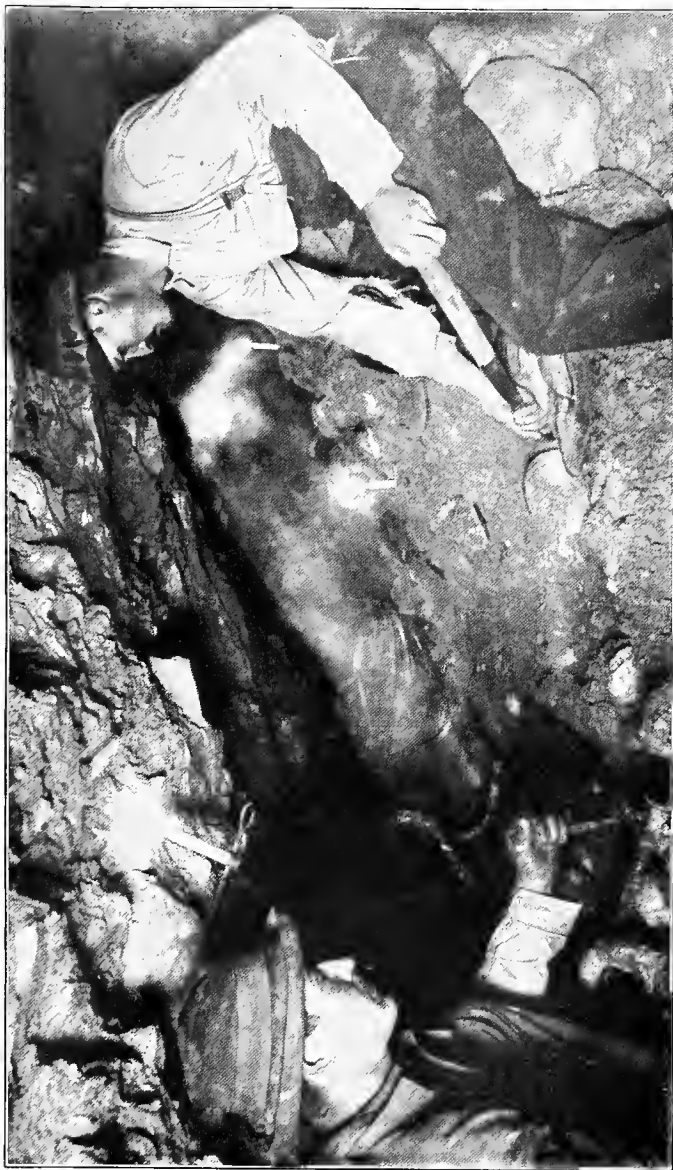
BILL STOPPED WHERE A COUPLE OF WORKMEN WERE BREAKING INTO THE SIDE OF THE DRIFT
